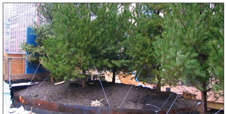
Not all green roofs are the same. At 101 Warren Street in downtown Manhattan, soil from Long Island Compost was used in an ambitious 101-tree green roof forest, with roof deck planters on several upper level floors.
